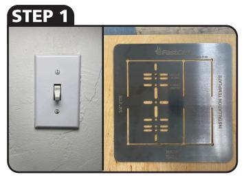
PICK SCREW ON PLATE AND FIND CORRESPONDING HOLE ON ETR 3/4 JIG
