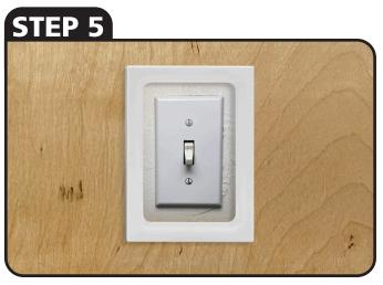
REMOVE JIG AND CUT TABS & INSERT ETR 34 INTO CUT HOLE
