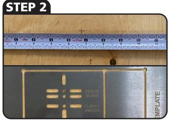
MEASURE AND MARK HOLE LOCATION AND ALIGN SCREW HOLE
